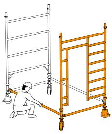
Position a temporary deck next to the diagonal brace. Fit the stairway between the master rung and the top cross member of the span frame. Ensure that the stairway claws are positioned outside the datum rivets on the master rung as shown.
